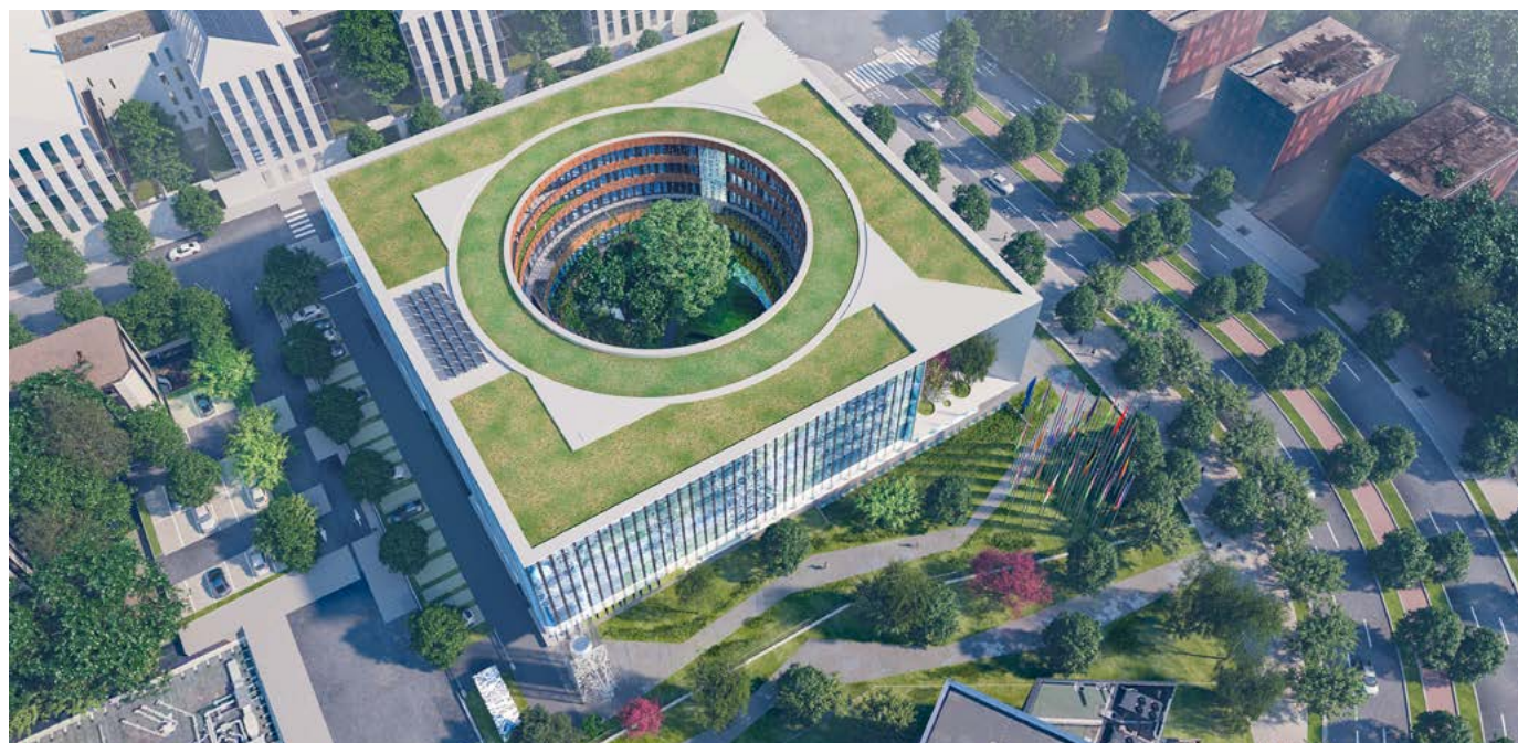
Aerial view of the future IARC Nouveau Centre. © ART & BUILD, architect s.a.
