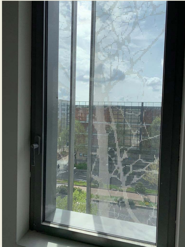
Outside view through the double façade system
