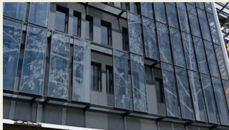
View of the South façade - Second skin under works
